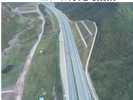
K87+900 处路基（半挖半填）恢复
