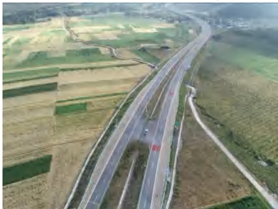
K90+000 处路基（填方）恢复
