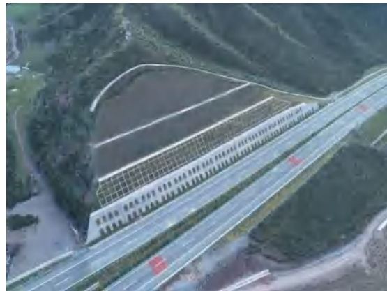
K84+200 处路基边坡恢复
